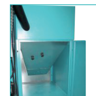
Pellet tank cleaning openings
