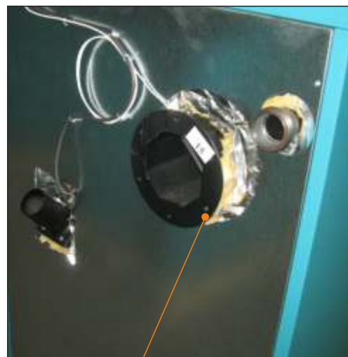
Flange for mounting fan
